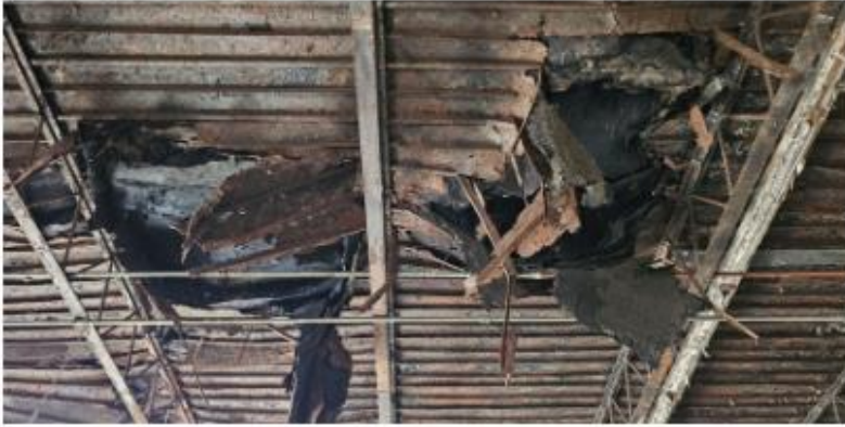
INTERIOR- ROOF STRUCTURE AND DECK CONDITION
