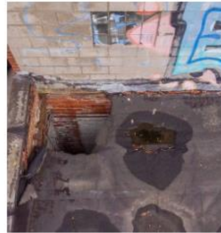
EXTERIOR- ROOF PENETRATIONS
