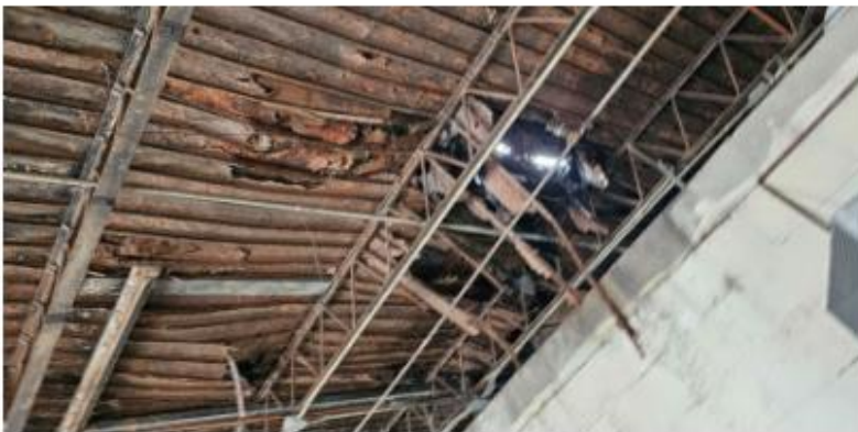
INTERIOR- ROOF STRUCTURE AND DECK CONDITION
