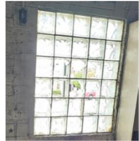
EXTERIOR- ROOF PENETRATIONS
