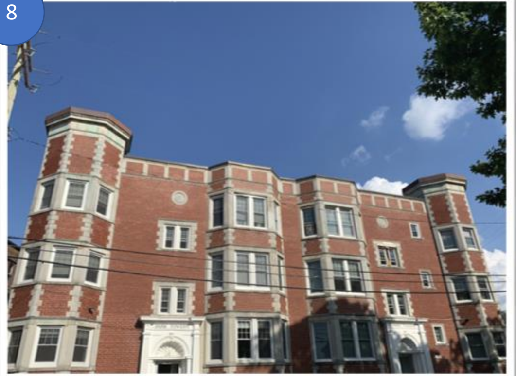
1415 West 112 St – Looking East
