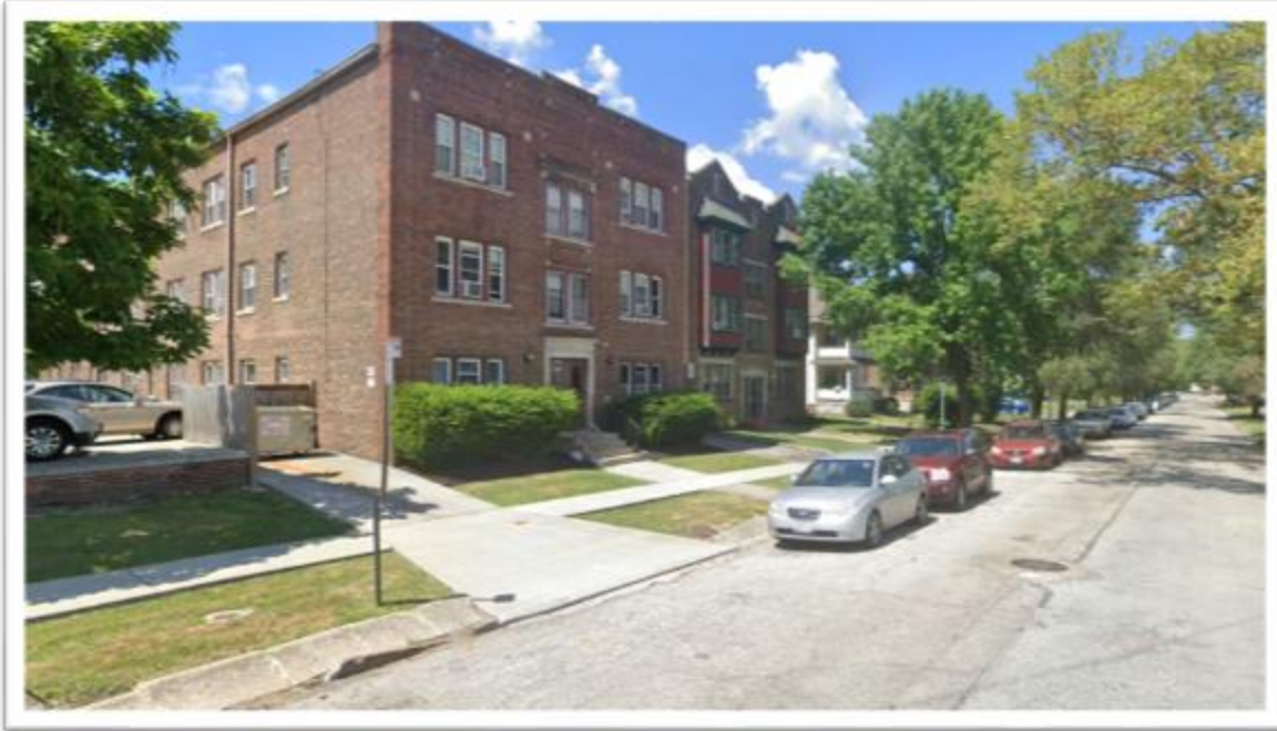
West 116 th St - Between Fruitland Ct & Clifton Blvd (2022, Google Earth)
