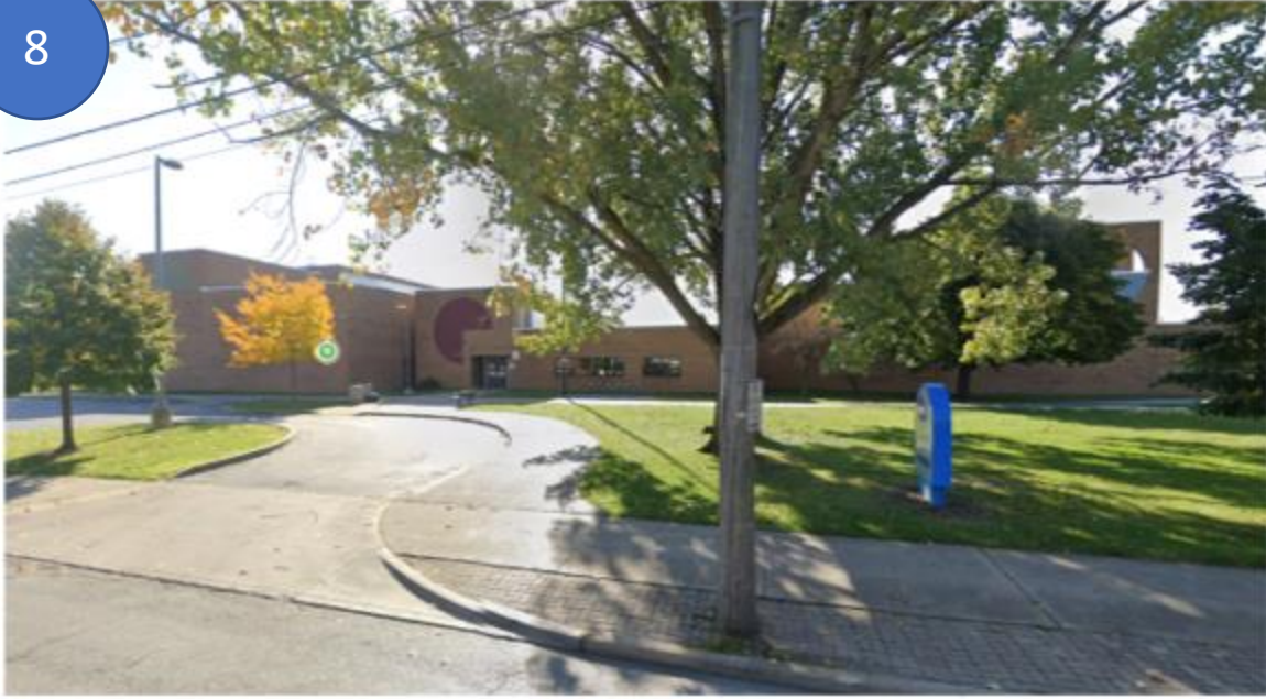
Zone Recreation Center, Lorain Avenue – Looking South 2022 Street View (Google Maps)
