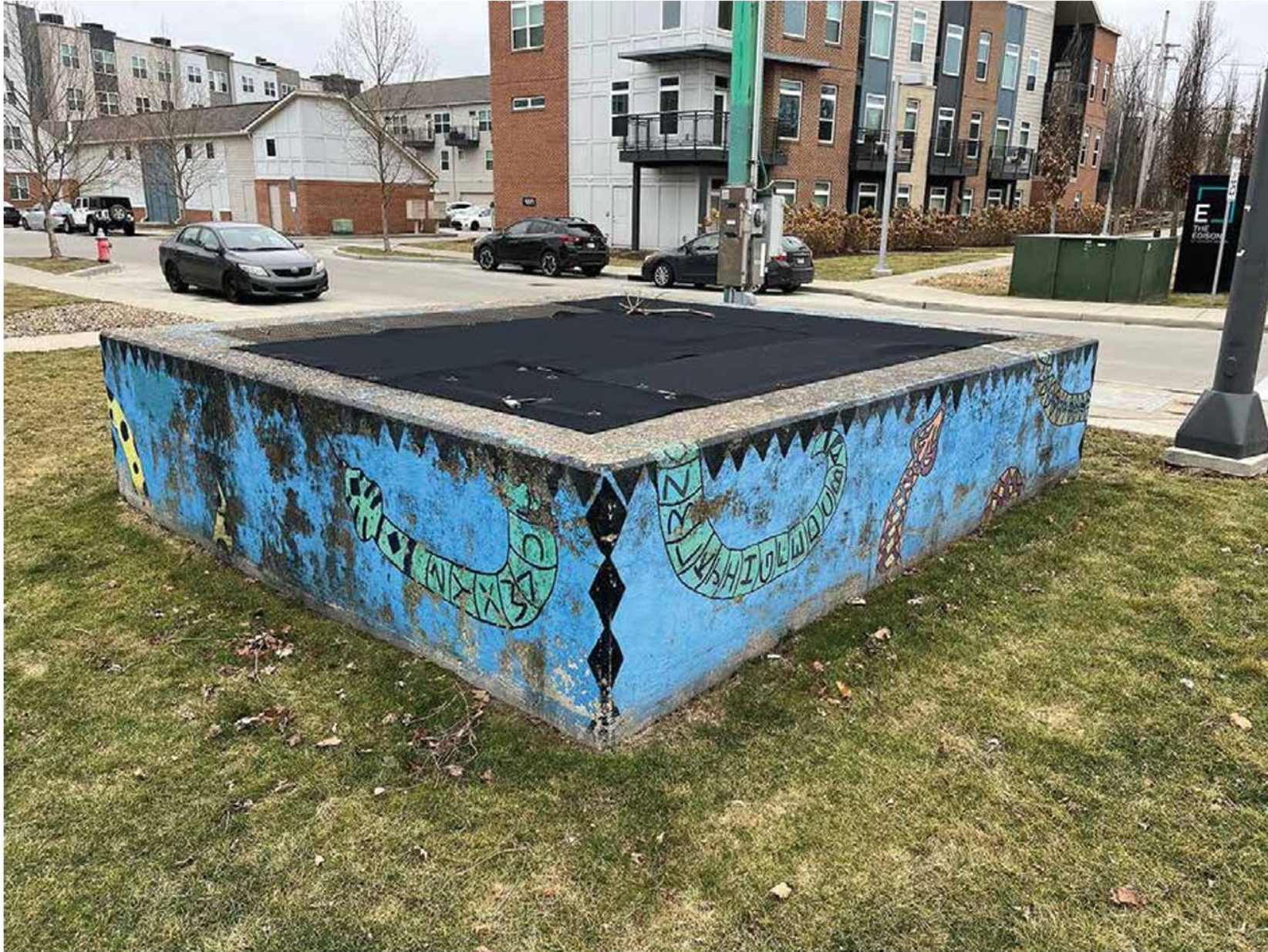
Close up view of current structure.
