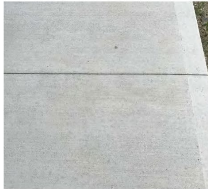
Broom Finish Concrete
