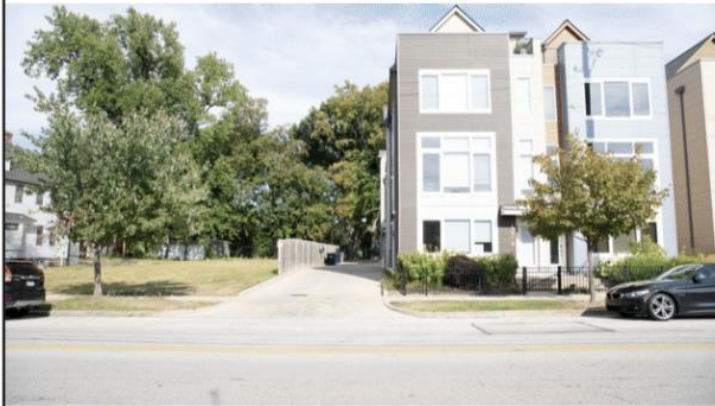
ADJACENT PROPERTY - 1561 E 118TH ST (SOUTH SIDE OF SITE)
