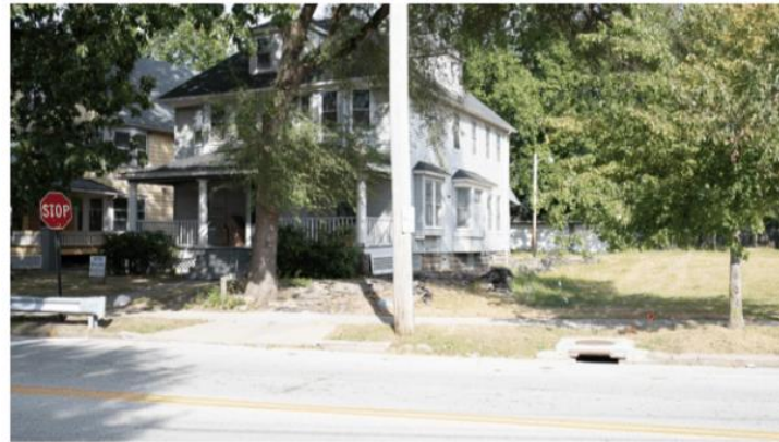
EXISTING PROJECT SITE- 1555 E. 118TH ST. CLEVELAND, OH 44106
