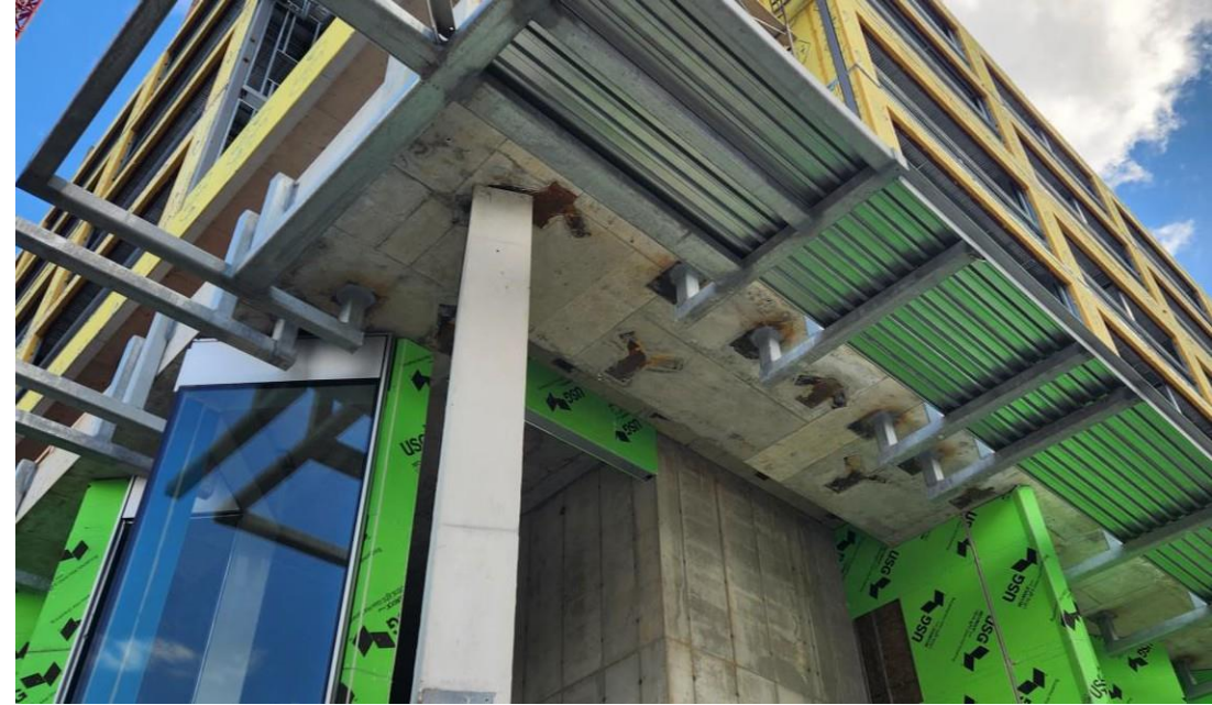
View of Glass Plenum Space Under Construction at Library Lofts Entrance
