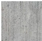
STANDARD CONCRETE - LIGHT BROOM FINISH
