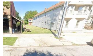
STREET SIDE PHOTO 3
