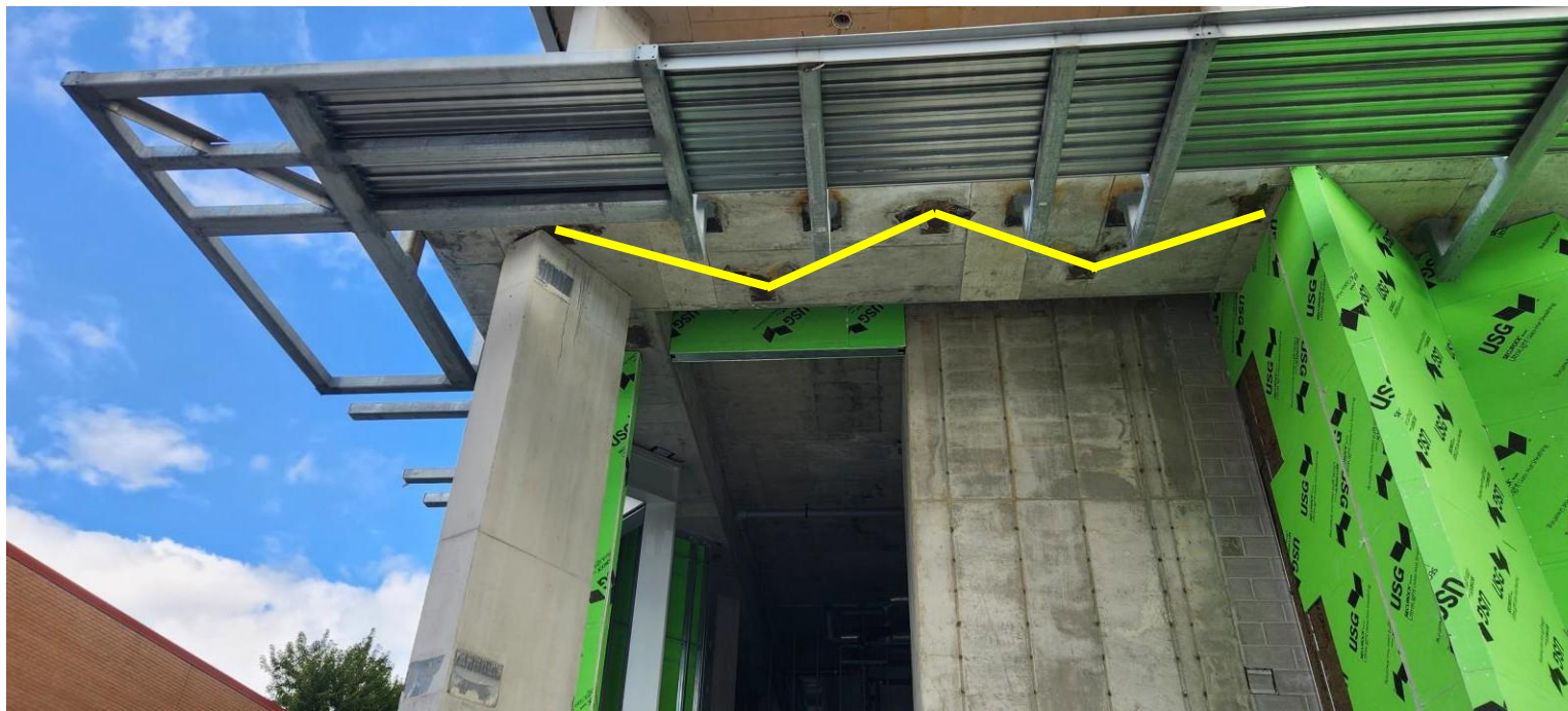
View of Glass Plenum Space Under Construction at Library Lofts Entrance
