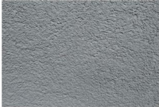
PT-3 7/8" 3-PART STUCCO W/ SAND FINE FINISH; BENJAMIN MOORE CHARCOAL SLATE FLAT
