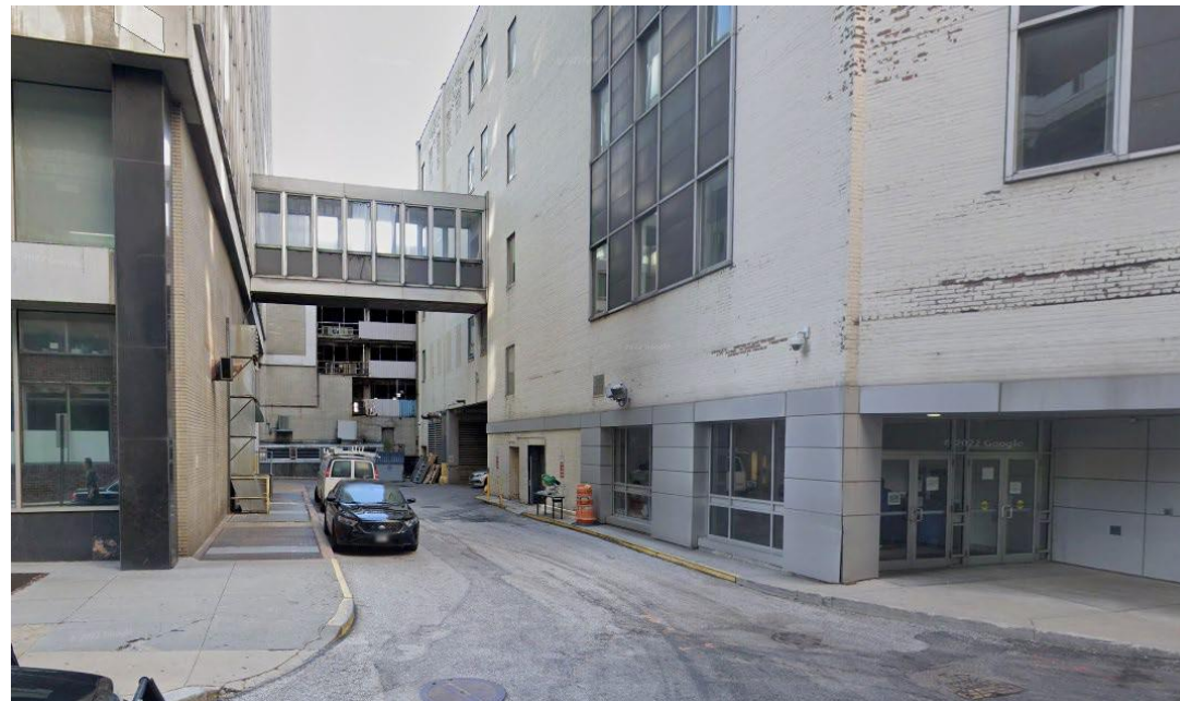
West down service alley
