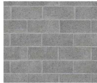
CMU Block Wall
