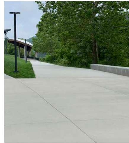
RECOMMENDED: Broom finish concrete
