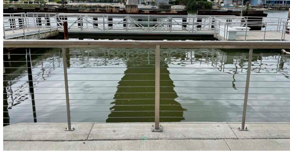
RECOMMENDED: Cleveland Metroparks railing - stainless steel and wood
