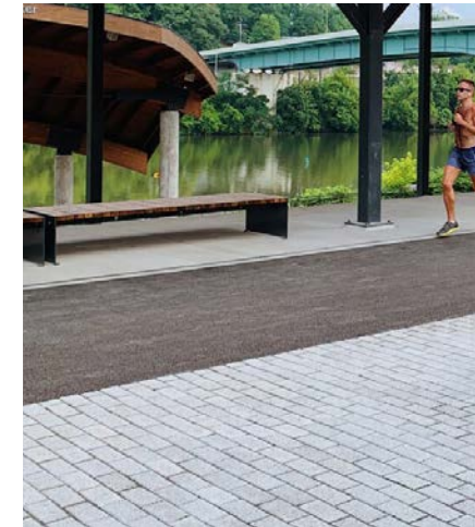
RECOMMENDED: Concrete unit pavers with square edges and minimal patterns
