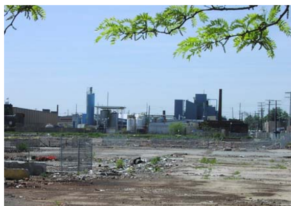
Brownfield sites are being re-envisioned as new industrial parks while funding is pursued for the necessary cleanup. [Midland Steel site in Cudell]
