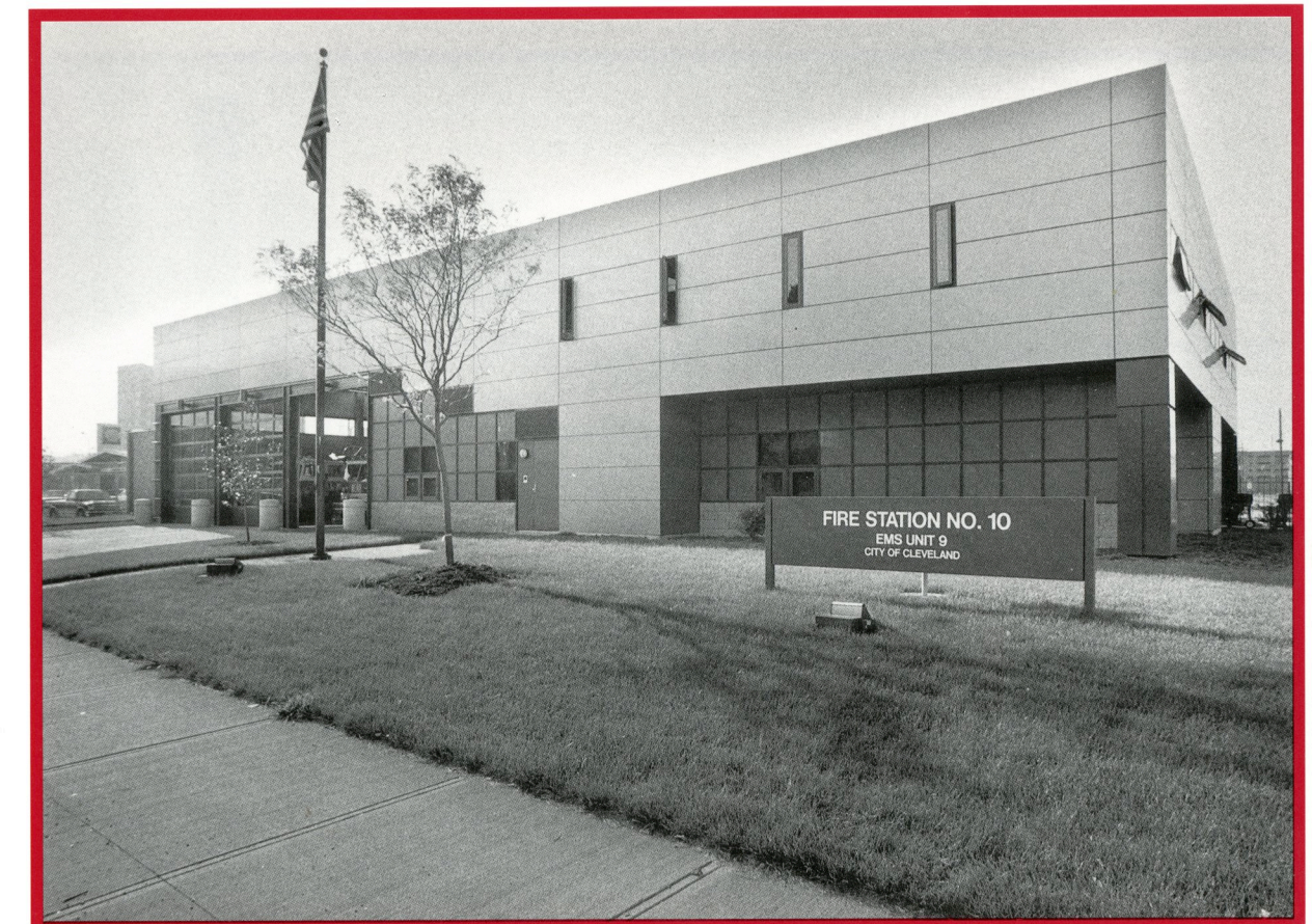
Fire Station #10 was built in 1986 to replace an outmoded 1875 facility located four blocks to the east of the new station. (LOCATION: East 101st and Chester).
