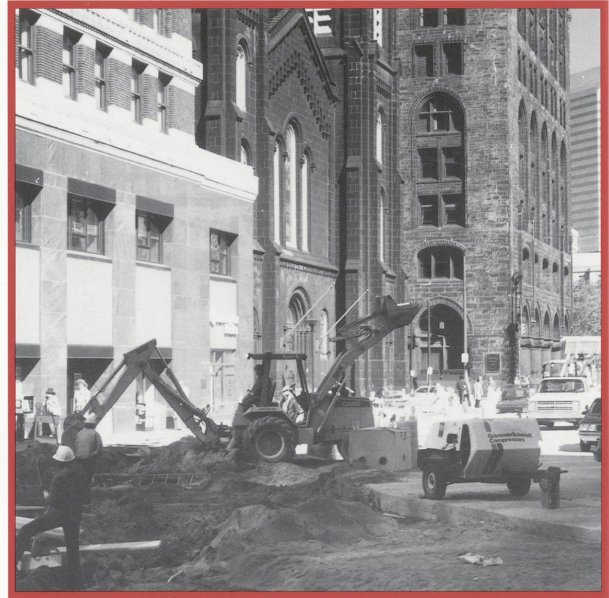
Utility Reconstruction on Public Square
