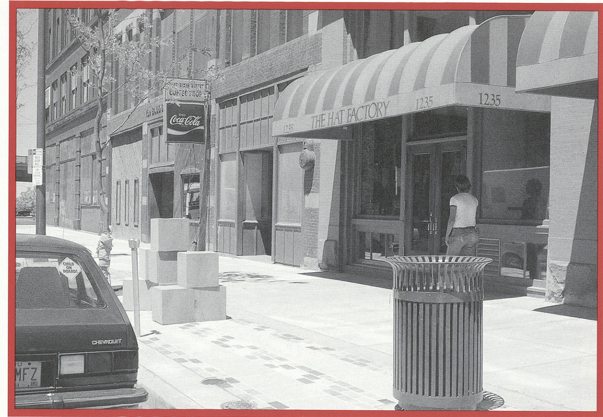
Streetscape Improvements on West 6th Street in the Warehouse District
